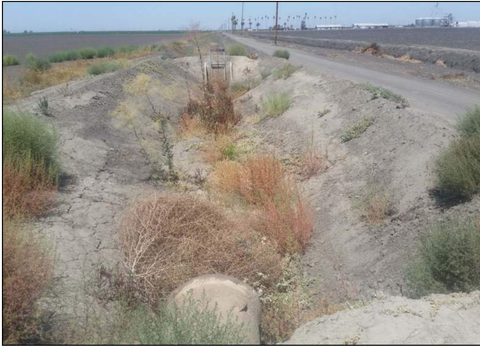
Figure 2a. Unnamed canal lateral, looking north.
