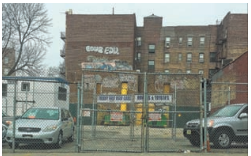
The proposed apartment building will occupy a vacant lot on White Plains Road and Thwaites Place. Community News Group/Sarah Valenzuela
