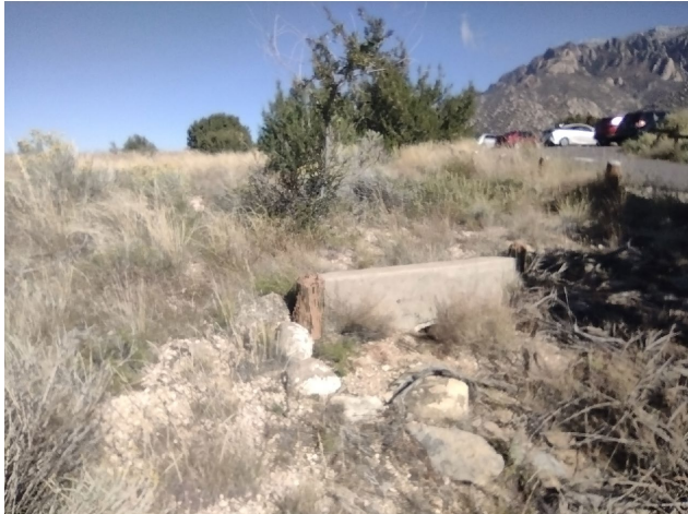
Photograph 9. Photograph of Northern Culvert at Site 3.
