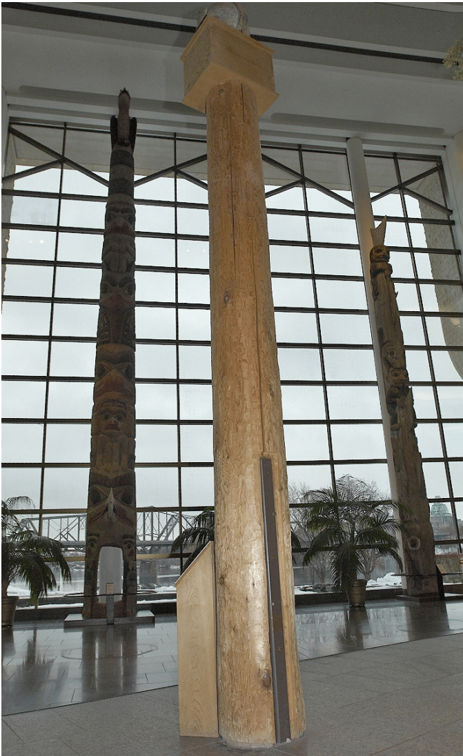
Figure 6. Rear of the White Squirrel support post at the Canadian Museum of Civilization, Gatineau, Quebec. The metal post is mortised fully into the cedar support post, and the base plate is hidden by the stone floor. Posts against the windows show plywood coverings over the base plate. Photo: Mylène Choquette, CCI (with permission from CMC).
