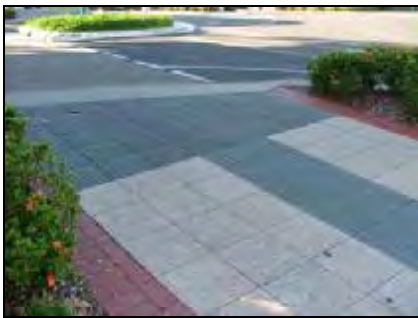
Tactile Indicators (dots adjacent kerb) and Directional Indicators (stripes) in the Cairns CBD (where concrete paving units are used to match footpath paving surface).
