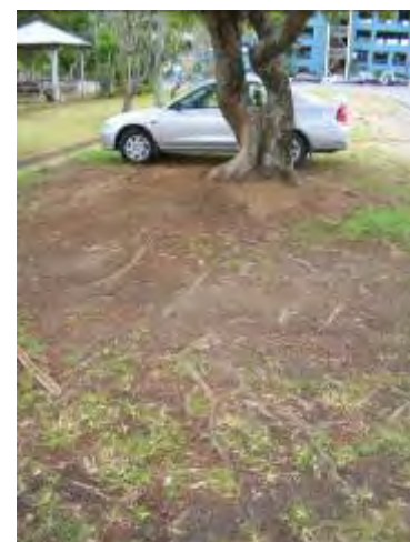
Tree roots have spread across the verge
