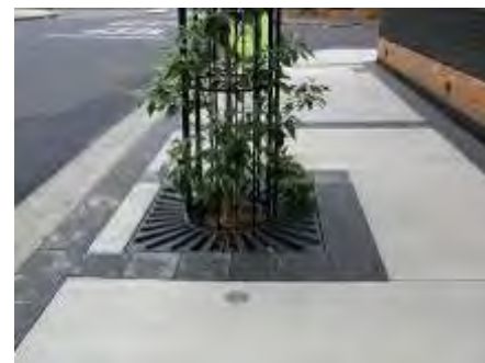
Tree grill and guard with aeration/water pipes
