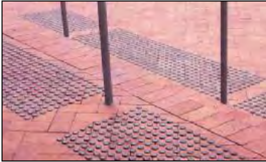
Tactile Indicators (where clay paving units have been retro-fitted with the product – see supplier details below).
