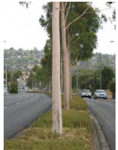
Root Directors have been installed in this median to minimise damage to infrastructure.
