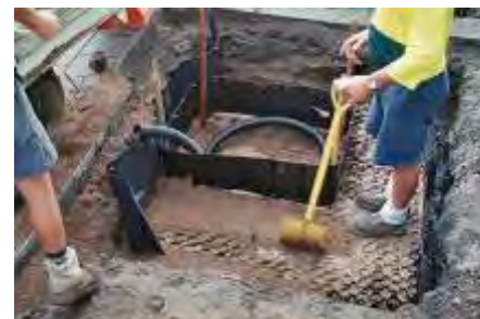
Root barriers installed over root cells with irrigation pipe
