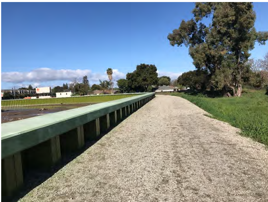
Figure 2-9. Example Sheet Pile Floodwall
