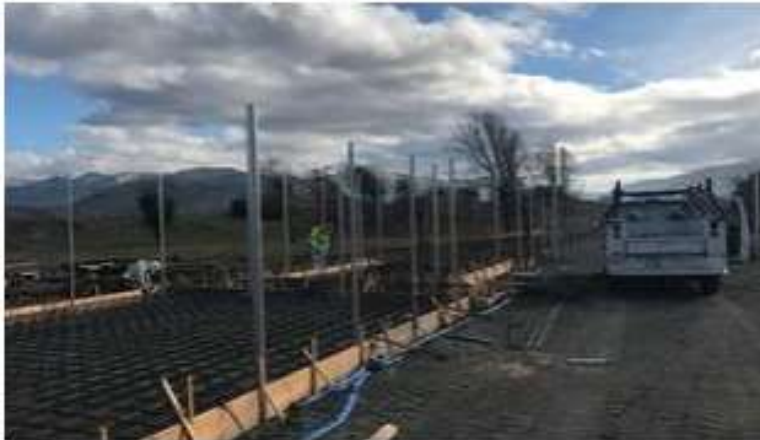
SFPUC - SUNOL NURSERY Sunol, CA (Started 2017 and scheduled to be completed 2018)
