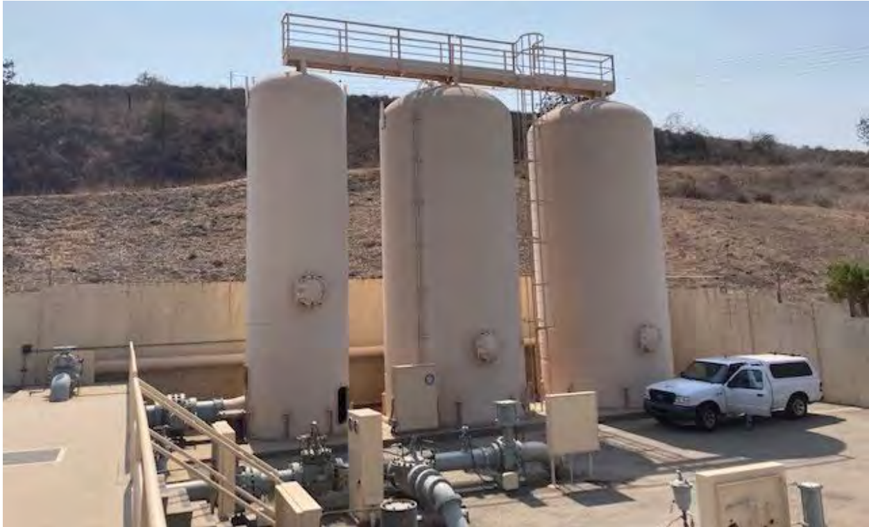
Figure 3 View of Surge Tanks, View Southeast
