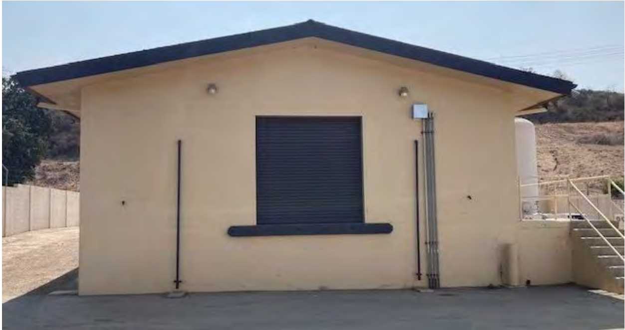
Figure 5 View of Control Building West Elevation, View East
