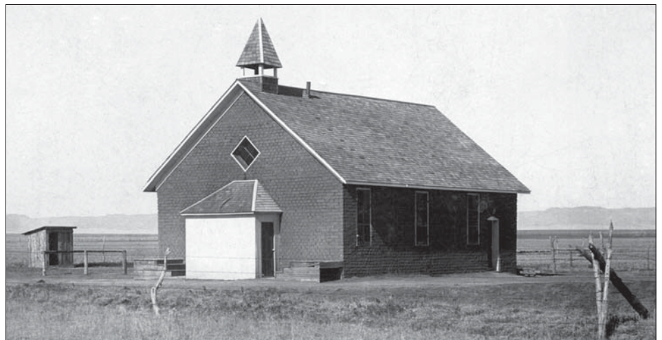
The Maxwell Christian Reformed Church, built with adobe bricks. Photo courtesy of the Archives, Calvin College, Grand Rapids, Michigan.
