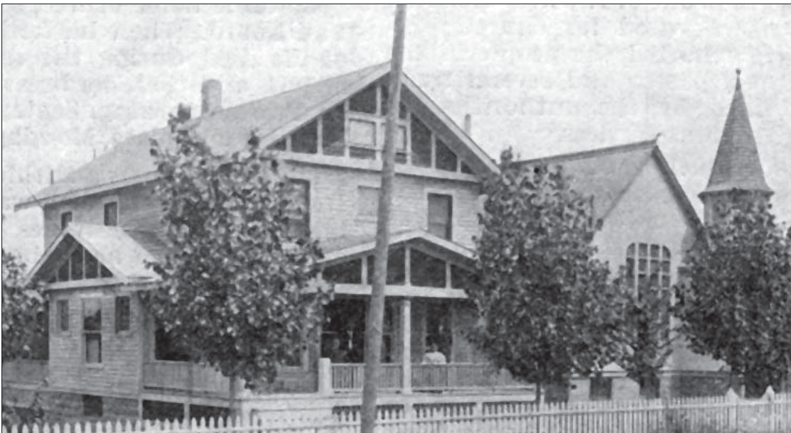
The parsonage of the Zillah Christian Reformed congregation was remodeled in the fall of 1911 by Johannes Daverman, father-in-law of the pastor, Cornelius Vriesman. Daverman established J. & G. Daverman, which was a long-time architectural firm in Grand Rapids. Image from The Banner, 12 September 1912, p. 576.
