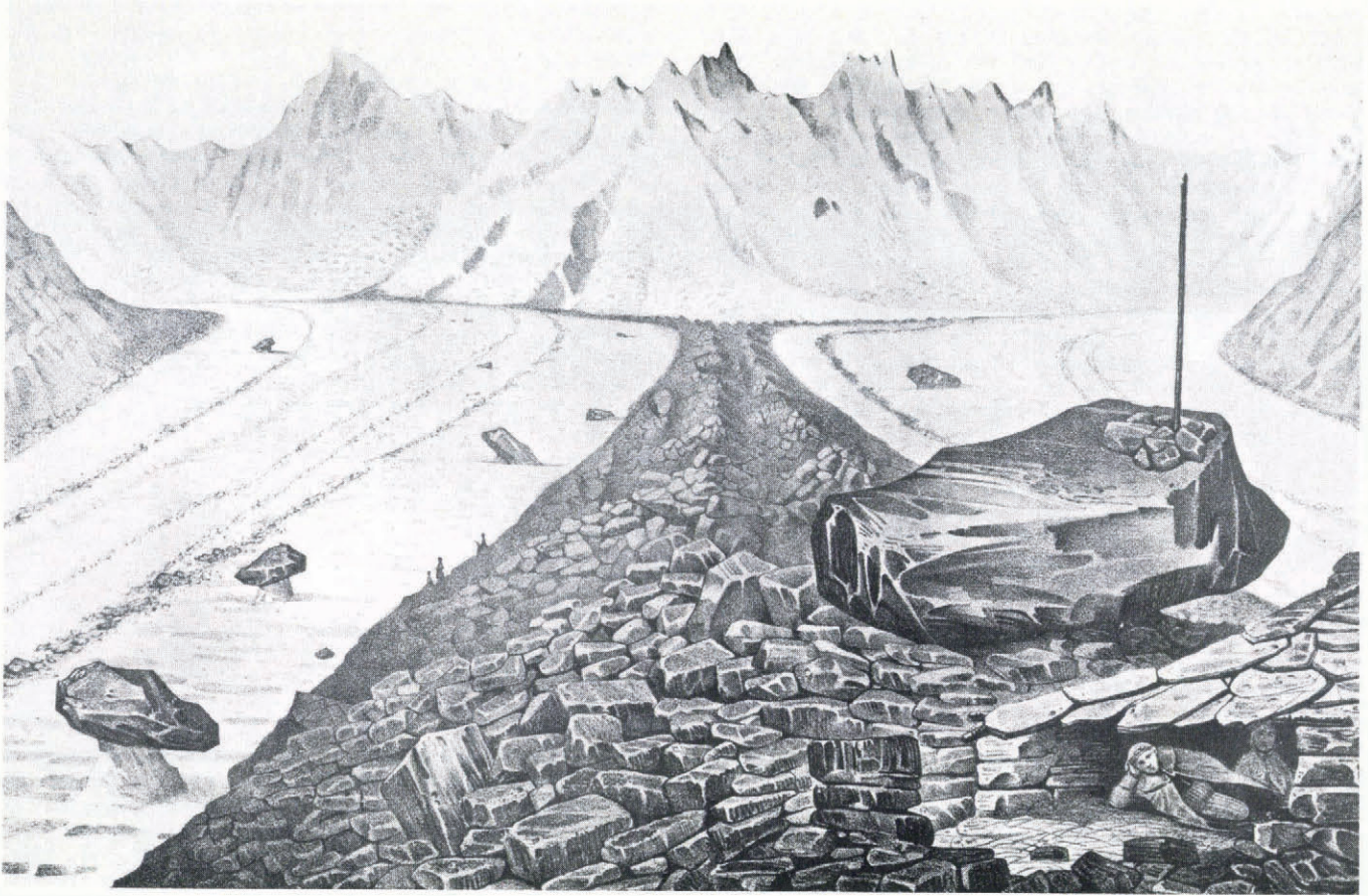
Fig. 1. Hugi's hut on the medial moraine of Unteraargletscher below the confluence of the Lauteraargletscher (left) and Finsteraargletscher (right). The hut moved from the foot of the rock Im Abschwang (centre) to this location in 13 years. This moraine was the site of Agassiz' Hôtel des Neuchâtelois , while he conducted research here in 1840. (With permission of the Rector, Université de Neuchâtel.)
