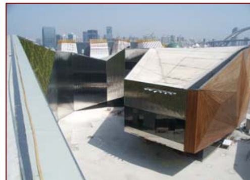
White Membrane Roof
