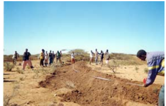
Photo 4: Measurement of earth bunds by project FFW labour
