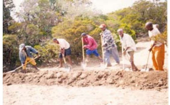
Photo 3: Construction of bunds using Food for Work Programme (FFW)
