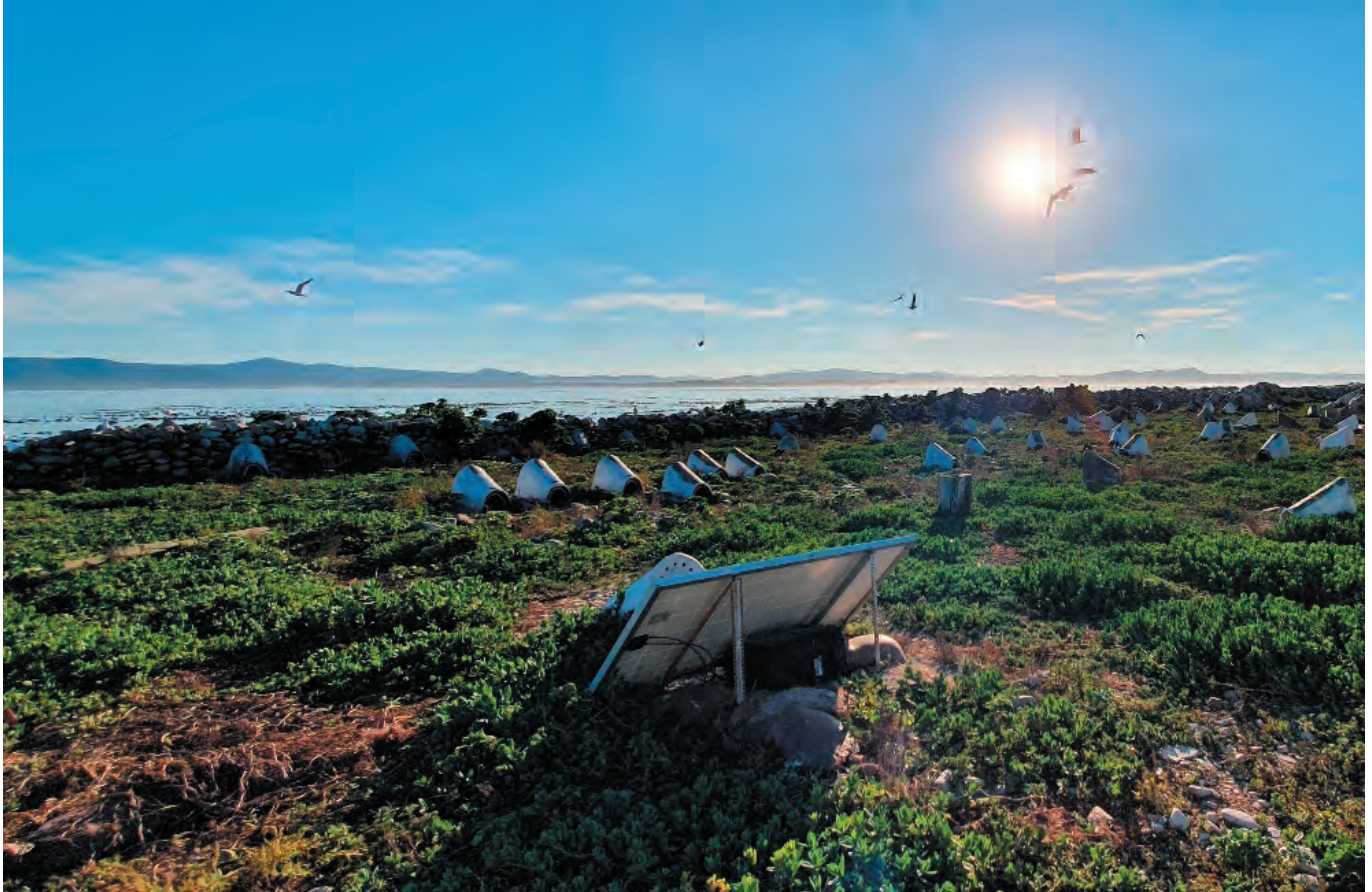
Figure 7.9: The solar panel located on Dyer Island to provide electricity to the buildings used for operations. Photo: D. Burger.
