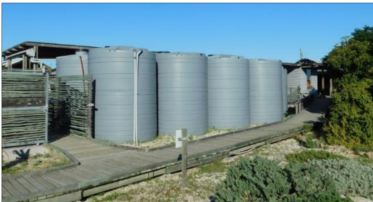
Figure 7.4: The Rocherpan rainwater system located in the office precinct provides water for staff and visitors (Photo L. Seabi).
