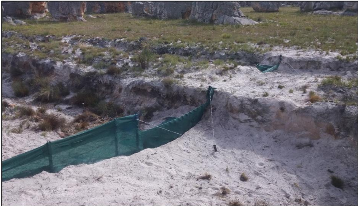
Figure 5.1: Perdevlei silt traps constructed as part of ongoing erosion rehabilitation efforts. Photo: Groot Winterhoek Field Rangers.
