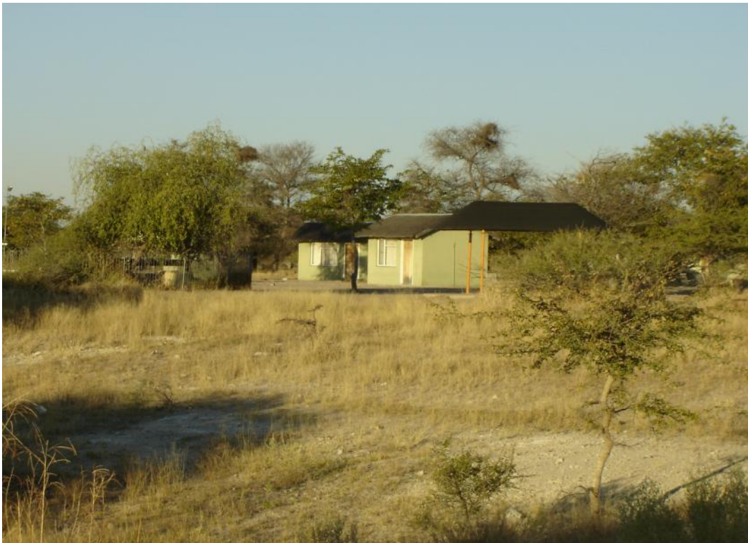
Photo 2: The Bays club at Mopipi dam
