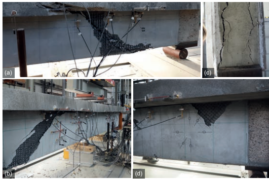
Figure 4: Failure mechanisms observed in this study: (a) crushing of concrete in the flexural compression zone; (b) rupture of tension strut; (c) transversal tension failure of the web at the underside; (d) delamination | graphic: Sebastian May, Alexander Schumann
