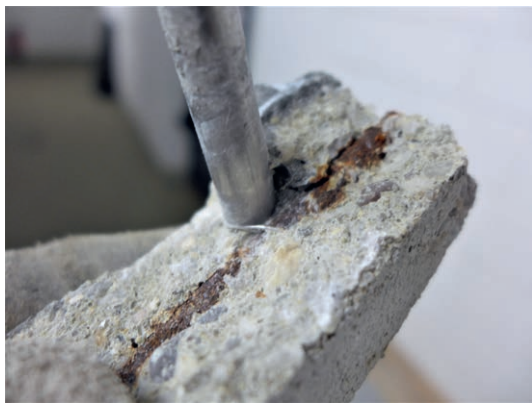
Figure 10: Refurbishment variant B after breaking the test specimen; the carbonated normal strength RC can be seen after removing of Pagel TF 10 layer; typical picture with very strong corrosion on the unalloyed reinforcing steel B500, mostly over the entire circumference and the entire length | photo: Jürgen Triebert
