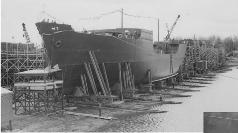
The USS Agawam, an Auxiliary Oil and Gas (AOG) tanker (Hull #3) under construction at the Port Cargill shipyard, 1943.
