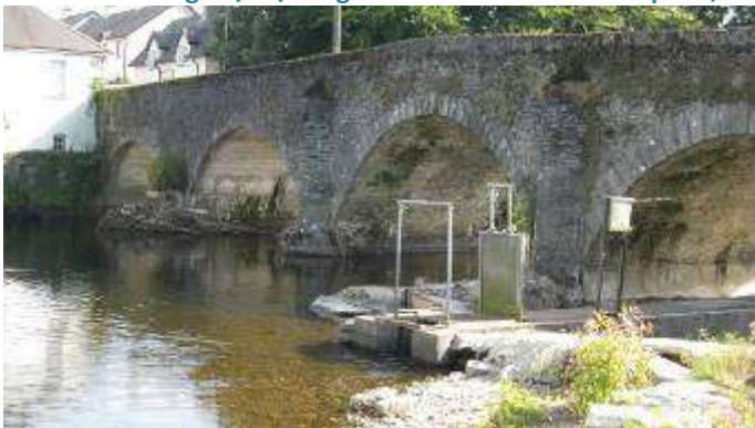
Clohamon bridge 2/09/10 from upriver showing debris, concrete reinforcing to 2 arches close to village(E)
