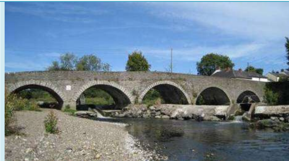
Clohamon Bridge 2/09/10: good cutwater feature to piers, already concrete repairs some loss of heritage value
