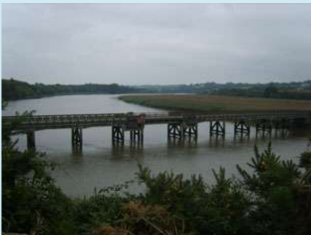
TOWNLAND DEEPS RIVER SLANEY RAILWAY BRIDGE, DEEPS NIAH 15703218
