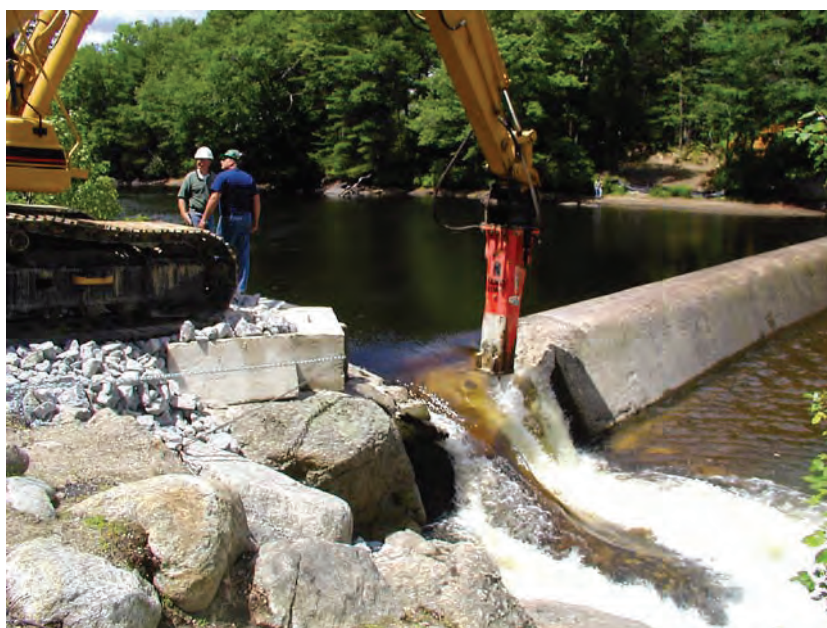
Removing a dam using an excavator with a hydraulic hammer attachment.
