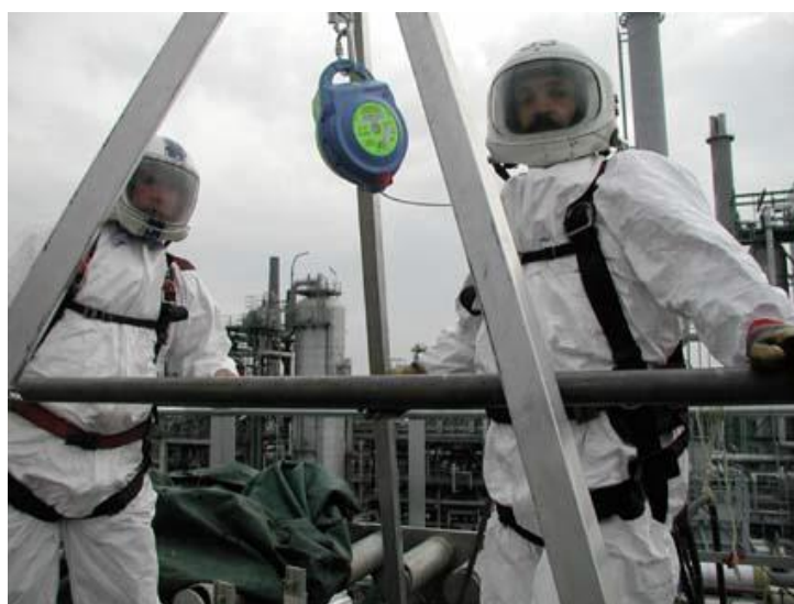
Figure 6: Operator with integral helmet and full breathing apparatus. The picture on the right shows the top of a reactor with fall arrest tripod.
