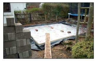
3" insulation laid over membrane
