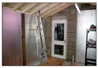
Insulation battened to walls
