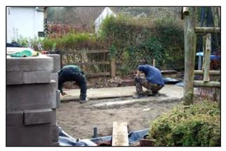
Concrete laid over insulation
