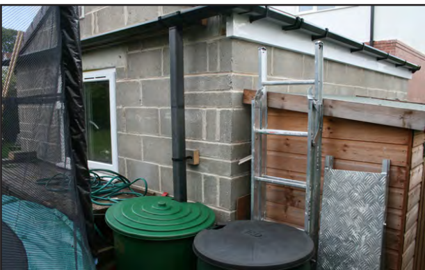
Rain water collection from fish house roof
