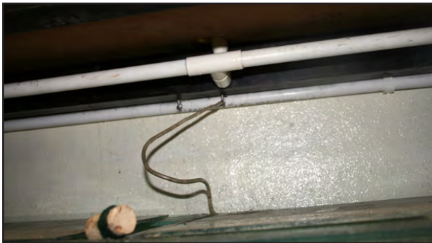
Underside of new centralised tanks
