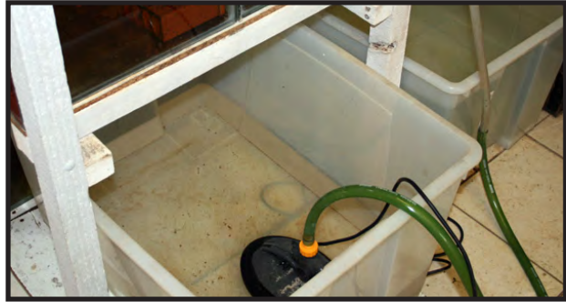
Rain water pumped to 30 gallon storage tubs before use in water changes.
