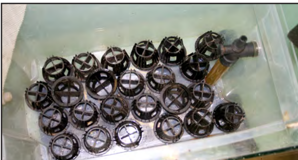
Step 1: Plastic filter media to create a void at the bottom
