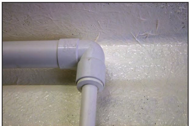
And stepped down through 22mm pipe
