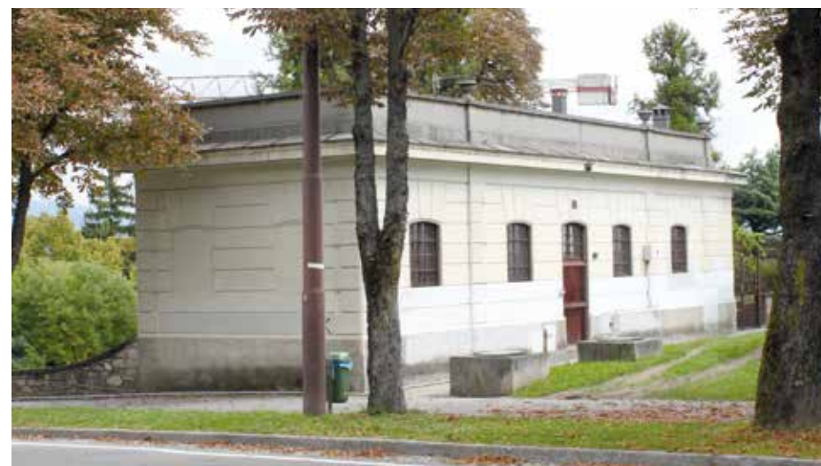
The pumping system now located above the tank of S. Agostino could pump 26,000 litres an hour up to the tank of La Rocca.
