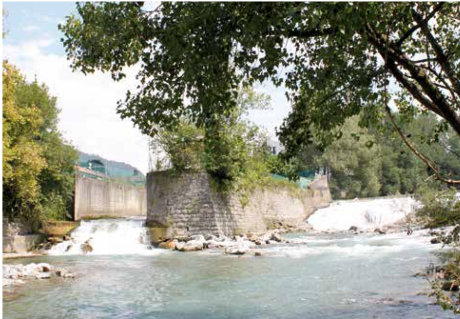
The inlet system that channels water into the Roggia Serio.
