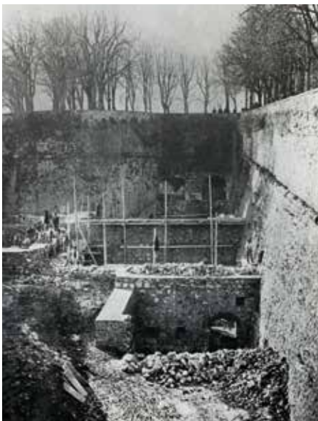
Work on the tank of S. Agostino in photograph from 1880.
