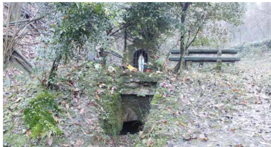
A second inspection chamber located in Via dei Vasi.
