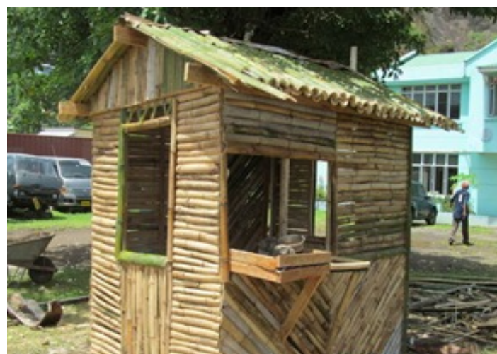
Building made of Bamboo
