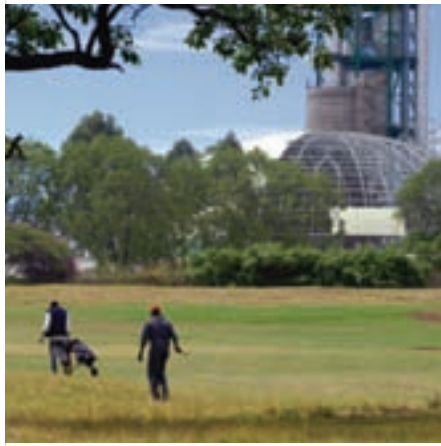
Cement plant in Zambia surrounded by a golf course
