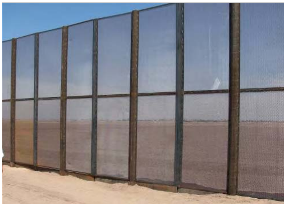
Figure A-2. Typical Primary Pedestrian Fence Design
