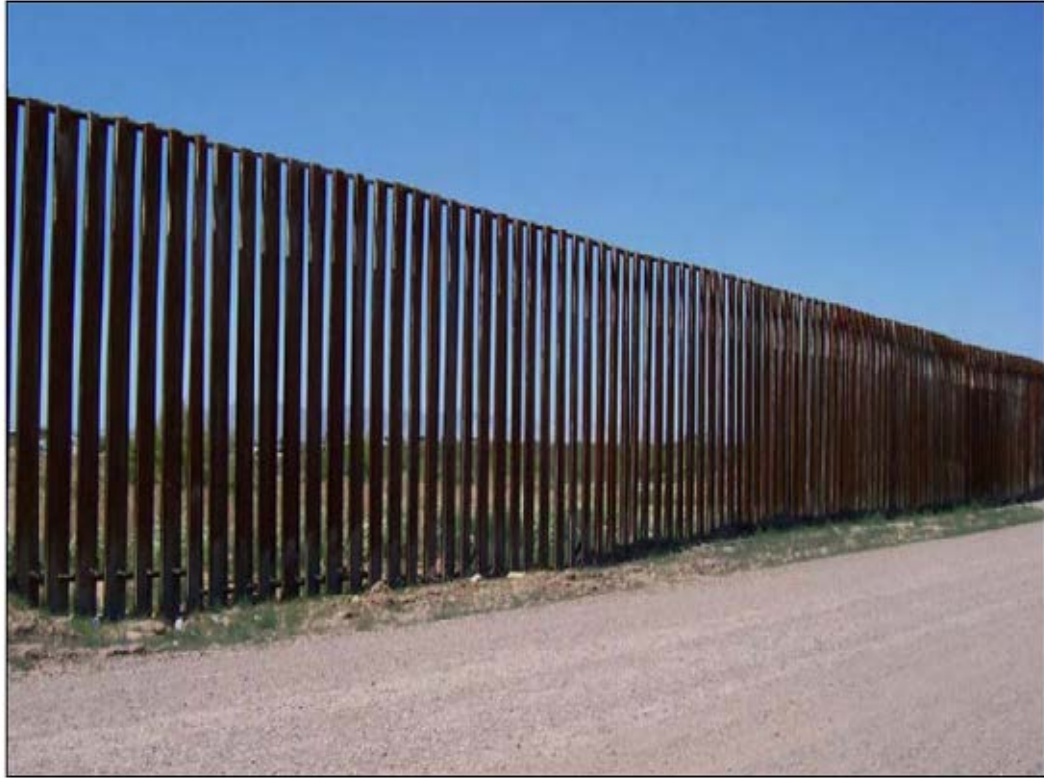
Figure A-7. Bollard Fence
