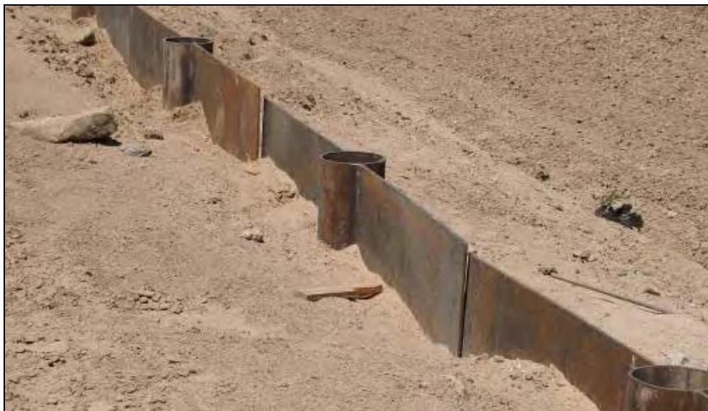
Figure A-1. Typical Primary Pedestrian Fence Foundation
