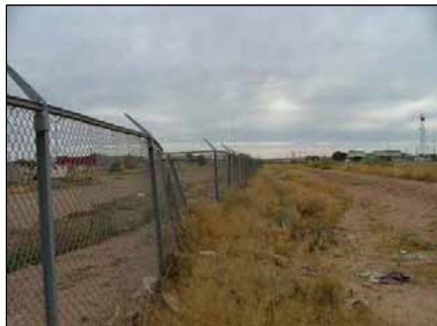
Photograph 1-2. IA Damage to TI
