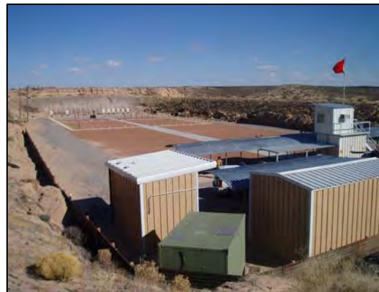
Photograph 1-2. Firing range section of the existing range.
