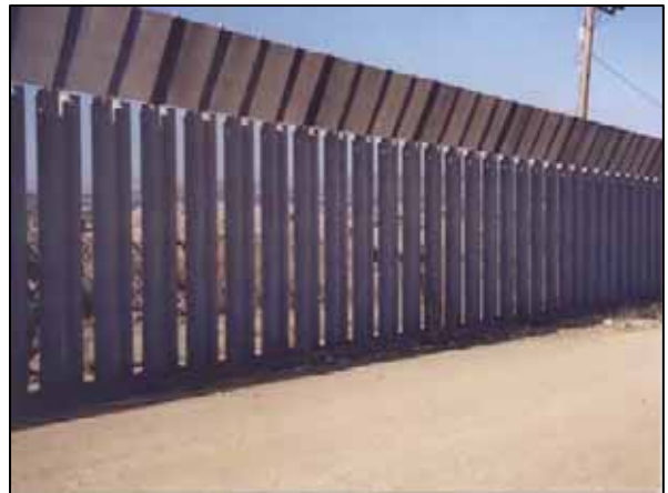
Photograph 2-3. Typical Bollard-style Pedestrian Barrier
