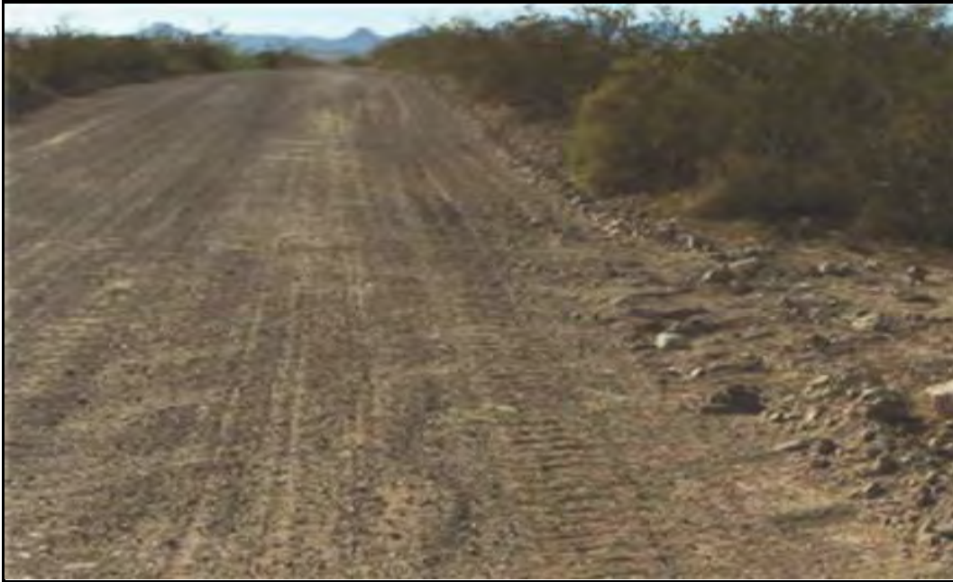
Figure C-5. FC-3 Graded Earth Road (Photograph)
