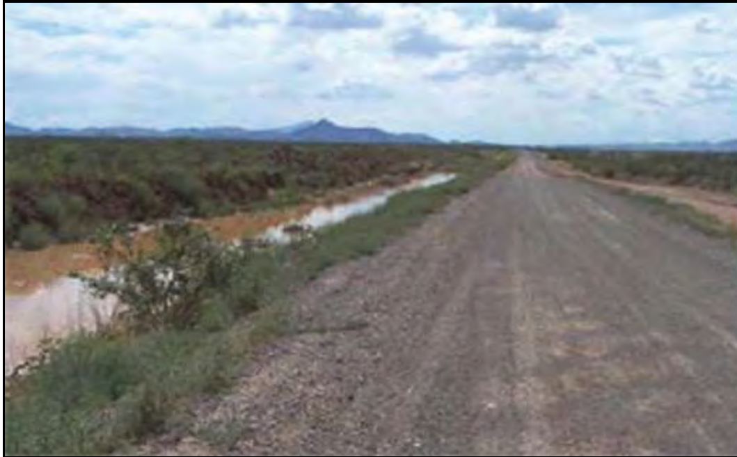
Figure C-3. FC-2 All-Weather Road (Photograph)
