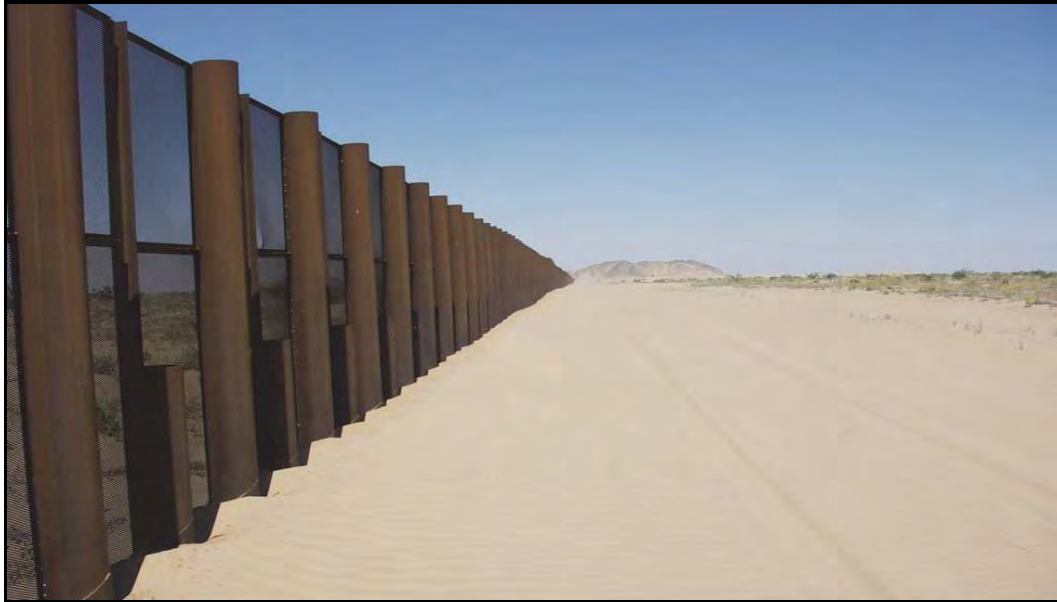
Figure C-9. FC-5 Sand Road (Photograph)
