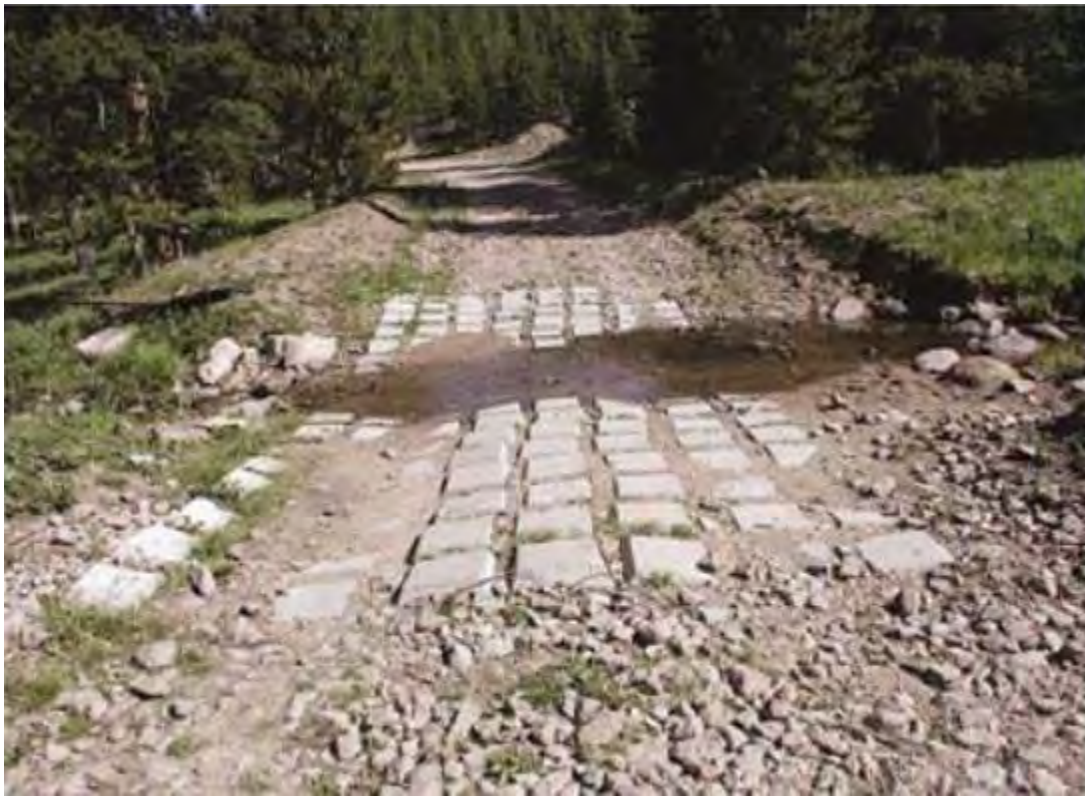
Figure 3. Low Water Crossing and Concrete Mat Example
