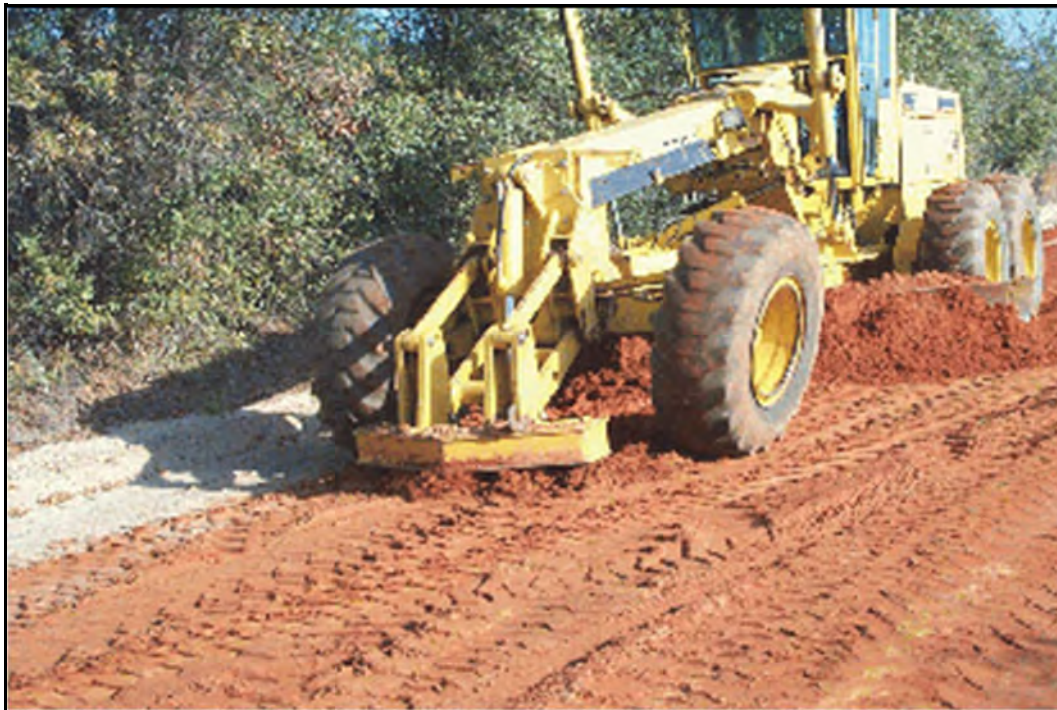
Figure C-11. Standard Grading Equipment
