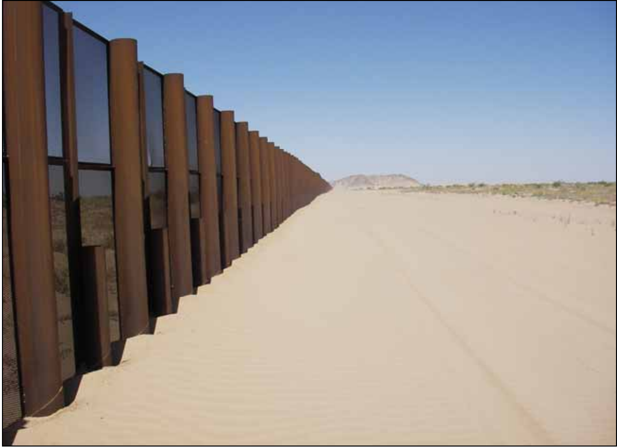
Figure C-9. FC-5 Sand Road (Photograph)
