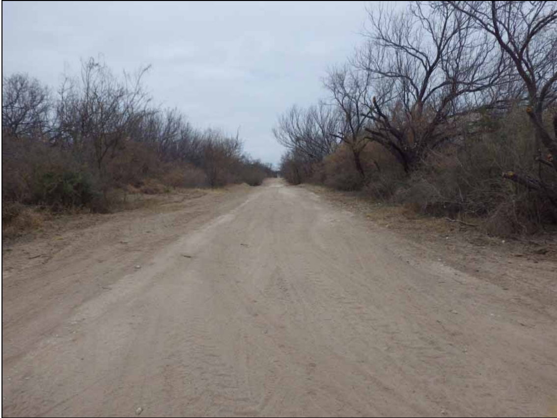
Figure C-5. FC-3 Graded Earth Road (Photograph)
