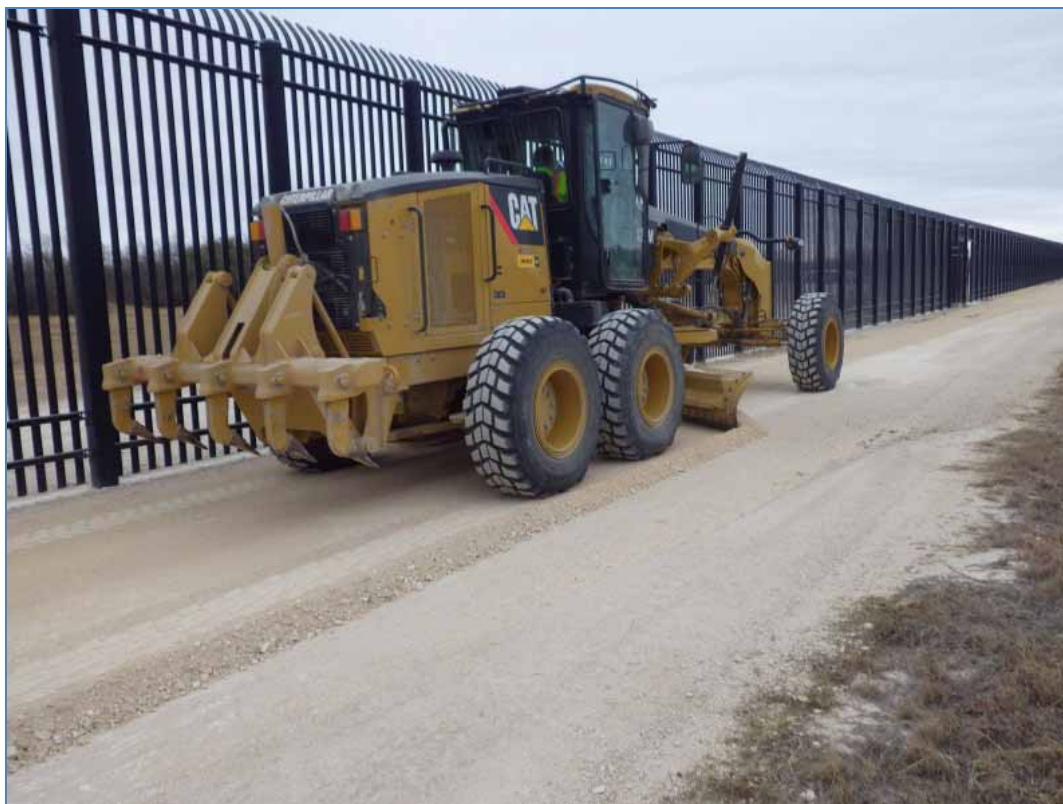
Figure C-11. Standard Grading Equipment
