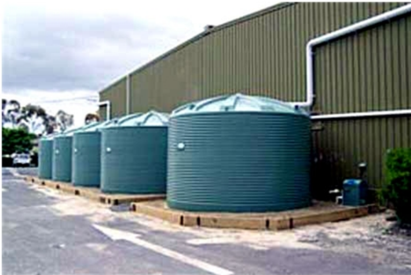
Figure 8a – Rainwater Harvesting in a Non-Residential Setting
