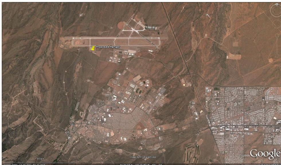
Figure 1 – Proposed hanger site on Fort Huachuca. The town of Sierra Vista is southeast. Image is about 17 miles across.
