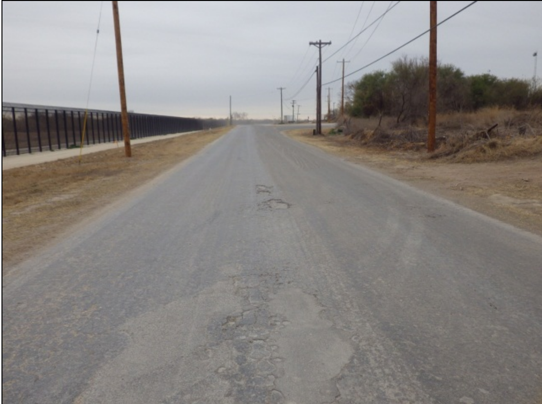
Figure C-1. FC-1 Paved Road (Photograph)
