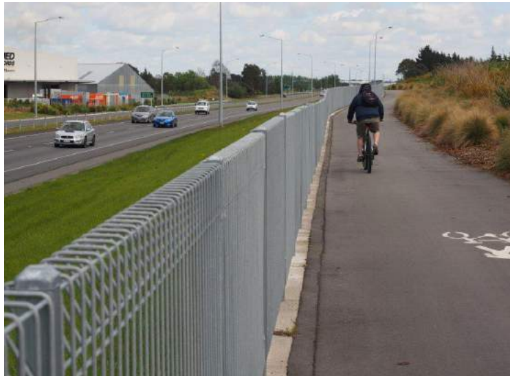
Christchurch Southern Motorway
