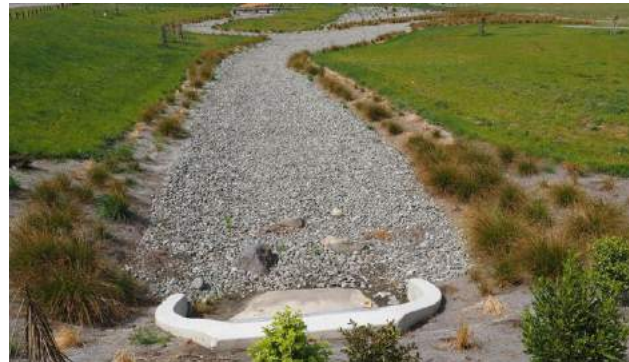
Carrs Road, stormwater basin
