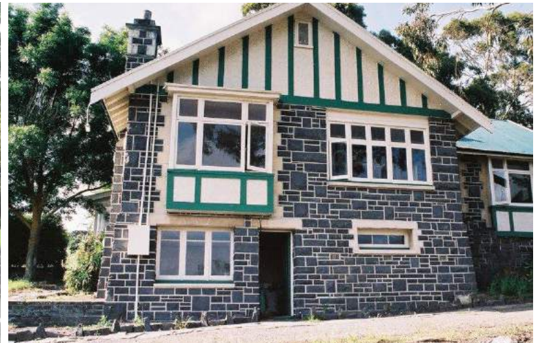
Quarry Managers House, Halswell Quarry Park
