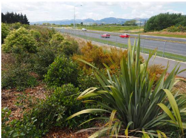
Christchurch Southern Motorway
