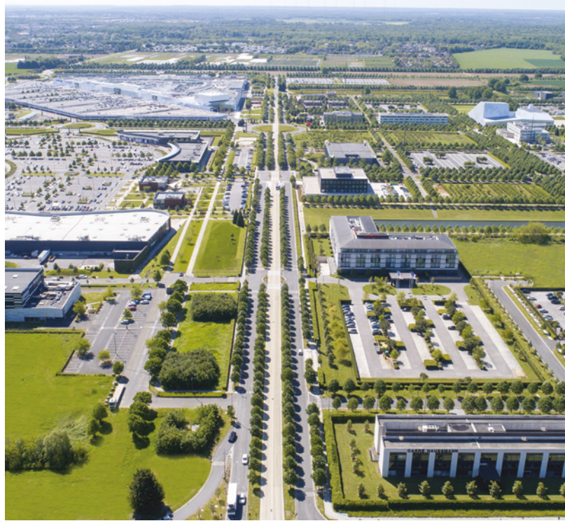
Urban Center Carré Sénart © Techniflight. Multiple Architects
