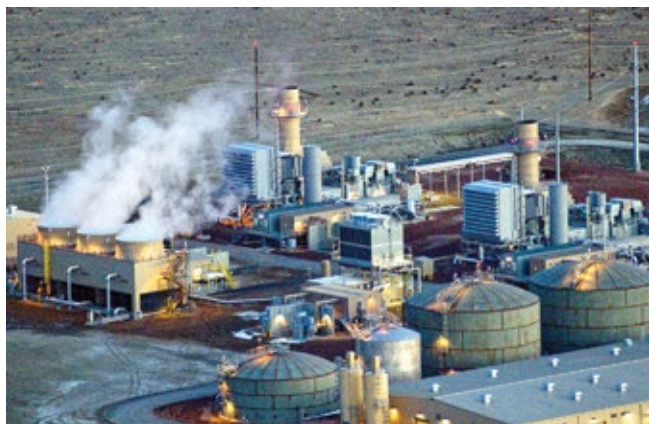
15. Pueblo Airport Generation Station produces up to 380 MW with its two LMS100 peakers (left) and two LM6000PF-powered 2 x 1 combined cycles (right)
