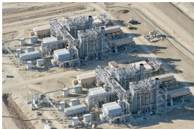
15. Pueblo Airport Generation Station produces up to 380 MW with its two LMS100 peakers (left) and two LM6000PF-powered 2 x 1 combined cycles (right)
