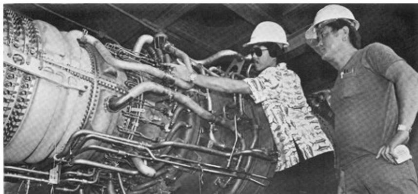
1. Wayne Kawamoto needs shades to protect his eyes from the reflection off the first LM2500 engine installed by Stewart & Stevenson in the US. The year is 1983, the place was Hawaiian Independent Refinery. Mark Axford remembers
