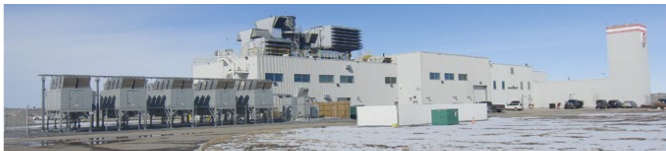
13. TCT opened its 220,000-ft 2 Airdrie custom depot in 2011. It is equipped with state-of-the-art engine test facilities. Note the GT inlet and exhaust structures on the building roof and the load banks to the left
