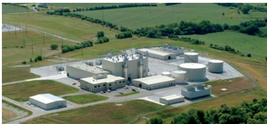
14. Terry Bundy Generating Station, equipped with LM6000s, stands out for its recognized safety practices
