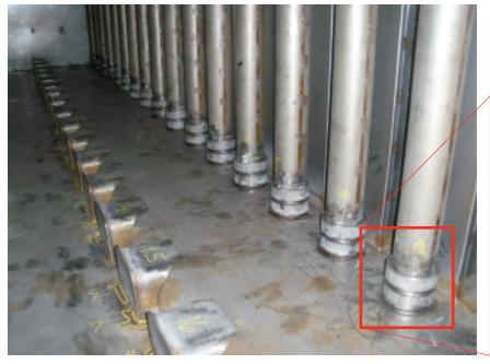
**11. Installation of the new guide sleeves** went according to plan and has eliminated the need for annual crack repair
