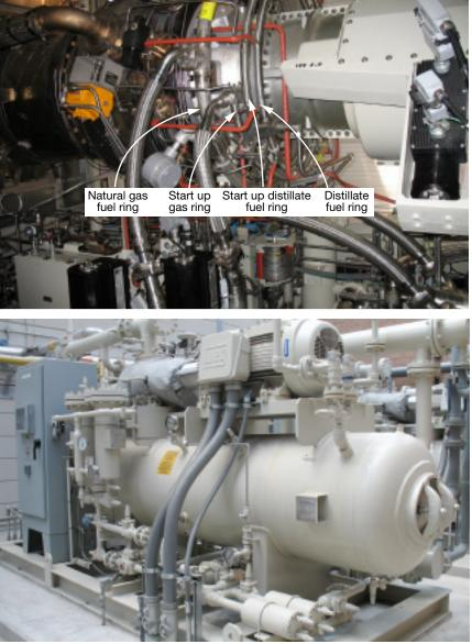
**3. Compression skid** boosts gas pressure from 40 psig as received to the 265 psig required by the Taurus<sup>™</sup> 60's combustion system. Three skids are installed (one a spare) to remove liquids, particulate
