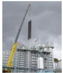
5. New HP evaporator module, located immediately downstream of the ammonia injection grid (refer to Fig 4), is lowered into place. The single HP superheater module also was replaced (left)
