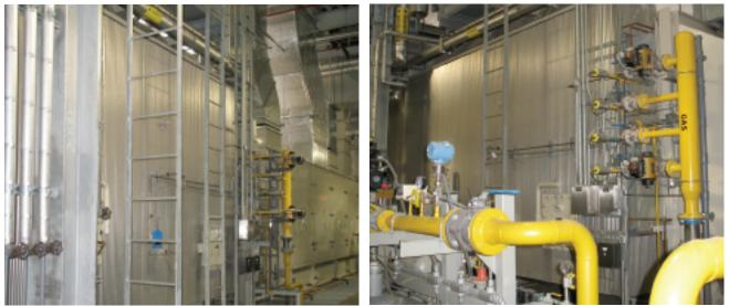
5, 6. Waterwall surface for HRSG is in the foreground of photo at left looking down at the Taurus 60 package. At right, duct burner and fuel skid are visible looking toward the rear of the waterwall section. Such tight spacing required locating catalyst beds and economizer in the vertical section shown clearly in Fig 4 but not here
