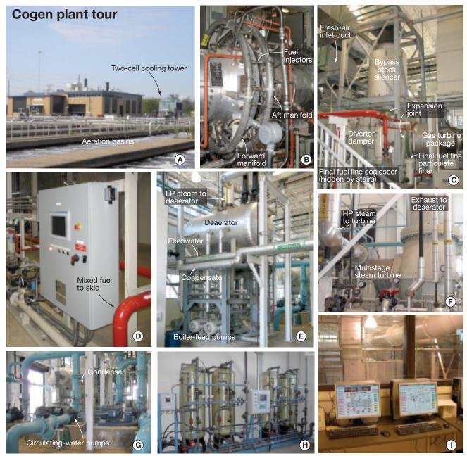
6. Cogen plant (A) tour begins at the gas turbine (B) and follows the exhaust gas flow into the HRSG (C). Fuel skid for the duct burner is in (D). Walking around the back of the HRSG (drawings in Fig 7) to the other side of the plant you find the deaerator and boiler feed pumps (E), steam turbine/generator (F), condenser and circulating water pumps (G), and makeup treatment system (H). Control room, one flight up off the main floor looks out onto the plant's major equipment (I)
