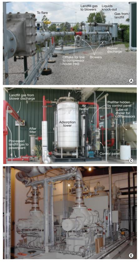
existed before the cogen plant, but it was upgraded as part of that project. The red spool piece in the middle of the photo, a tee, was added to direct landfill gas, previously flared, to the adjacent compressor building and treatment system where the green gas is cleaned-up before being piped to Bay View. Project engineer for this work was Mike Kemp of HCS Group Inc, Houston, a subcontractor to Solar Turbines.
