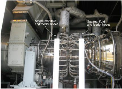
**2. Combustor arrangement** reveals one steam and one gas manifold. Steam here is for  $NO_x$  control
