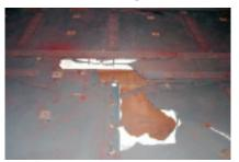
**3. Duct-liner damage** is relatively common in HRSGs required to cycle daily
