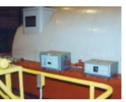
3. Condition monitor identifies any source of excess temperature
