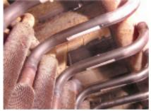
**10. Jumper pipes** connect header to fifth row of tubes after removal of the first four rows
