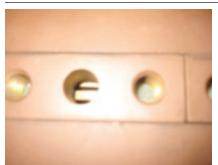
**17. Inspection via ventilation holes** in the wedges is possible on direct ventilated fields
