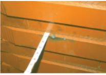
**14. Significant core damage** above could be overlooked by the untrained eye
