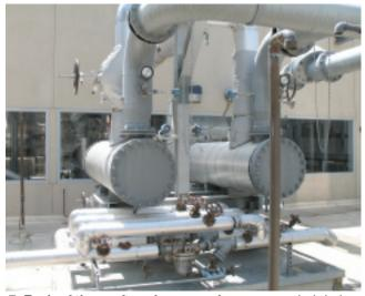
**7. Each of the rooftop dump condensers,** needed during process upsets, is capable of condensing all of the steam its dedicated HRSG can produce with duct burners off
