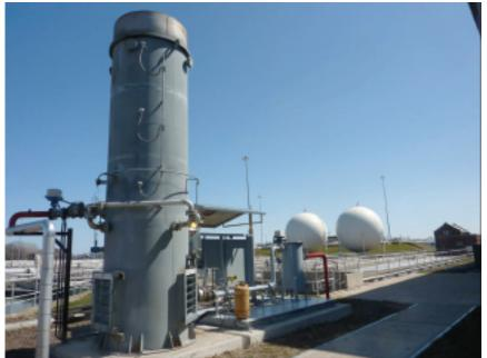
**4. Gas produced** in up to six anaerobic digesters flows from the spherical storage tanks highlighting the photo to the gas blending and compression station a few feet from the powerplant. Flare in the foreground is available for use when upset conditions dictate
