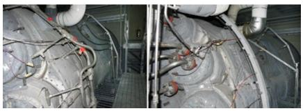
**1. Plant personnel** redesigned and replaced the original instrument wiring system (left) with one that provides more robust support and protection (right)
