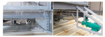
1. Original location of evap-cooler pumps is shown at left, new location at right
