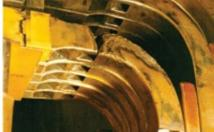
**4-6. Generator condition monitor** is very sensitive and will pinpoint the location of minor core overheating (left and center) and will easily detect at a very early stage any major damage (right)
