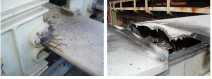
**6. Blown non-seg bus** at right is rare, but it happens; at left, damage caused by insulation break-down
