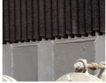
**4. Qinling's indirect-cooled ACC** features nominal 50-ft-long finned tubes at the base of the natural-draft tower. High-purity water circulates through the closed-loop cooling system
