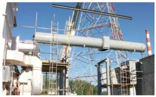
8. Circular non-seg bus has rigidity to facilitate transport and crane lifts
