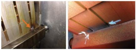
**1-16. Hot spots** are created because of poor contact surface at the core ends where current is transferred from the key bars into the laminations
