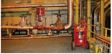
4. Corroded and misaligned steam pipe
