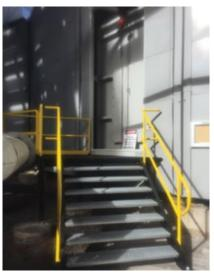
**3. Generous access** was provided at the door entry along with a temporary blank panel to muffle noise
