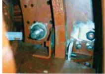
**1-15. Key-bar currents** want to connect through three parallel paths: core flange, core laminations, and frame components. OEMs have tried to bridge these currents via shunting straps and silver plating as shown
