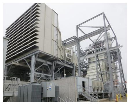
**1, 2. First 7FA.05** in foreground above exhausts through a heat-recovery steam generator which supplies the grey market D11 steamer below
