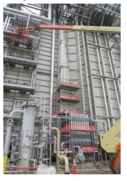
**5, 6. SCR ammonia system** reflects latest design. Blowers at left direct air to the heaters used to vaporize aqueous  $NH_3$  (left). Delivery system assures proper distribution of reagent to the catalyst bed (right)
