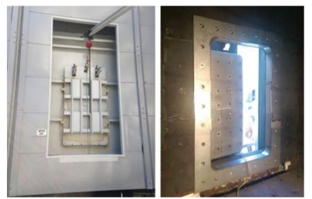
**2. The new door** required a trolley system for removal/replacement (left); door interior is at the right
