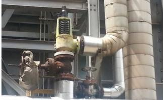
**11. Locking device** to prevent closure of block valve when steam system is in operation appears to be missing. A proper drain line at a low point in the steam vent system also seems to be missing (left)
