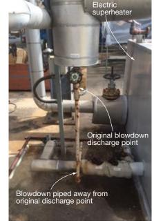
**1. Blowdown discharge location** for Effingham's auxiliary boiler was moved to prevent steam entry into the electric superheater
