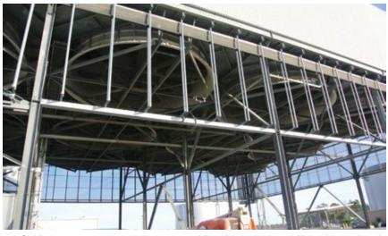
14. Caithness screens are shown retracted (front) and deployed (right side and rear)
