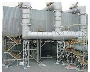
**18. ACC serving the 1 × 1 F-class** combined cycle at CCC Saltillo in Mexico currently operates with a combination of sheet-metal wind walls and 60%-mesh windscreens
