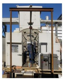
**3.** Collector rings are heated in oven (foreground, right of center), removed from oven, attached to chain-fall, lifted, and trolleyed to the generator
