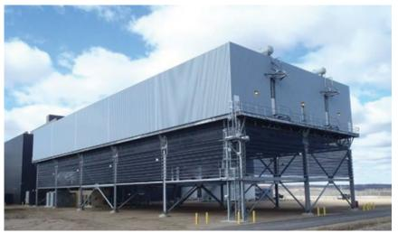
**9.** North Battleford, a  $1 \times 1$  combined cycle powered by a 7F.04 gas turbine, relies on perimeter screens for its ACC
