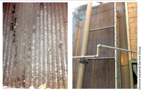
**11. Open-air heat exchanger,** severely fouled (left) was restored by  $CO_2$  blasting (right)
