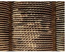
5. The tightly packed LP tubes are subject to both corrosion and fouling by ammonia salts
