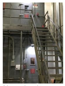
5. Low-cost, low-maintenance package door windows allow O&M personnel to assess interior conditions before entering a potentially hazardous situation
