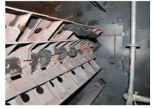
**4. A short flight** could show locations of burner-tip coking.
