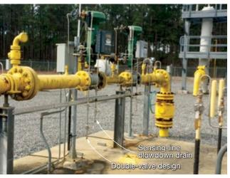
**4. Sensing lines** for fuel-gas-train control valves were equipped with drains and double valves to mitigate freeze-up in winter
