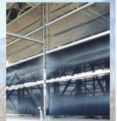
Top: Wind deflection screen Bottom: Wind and dust control fence showing integration of a doorway and conveyor
