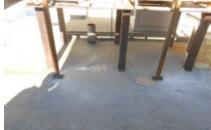
2. Legs supporting trolley system were bolted to the concrete pad to stabilize lifts
