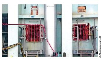
**7. Lower hatches for superheater** and HP evaporator access during outages. Temporary barricades are installed and lines for air, welding, and electric are secured
