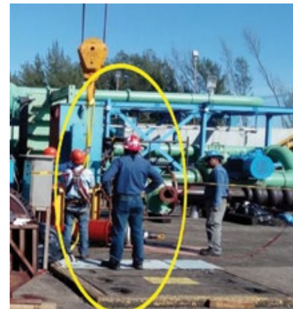
2. Safety watcher monitoring proper crane use
