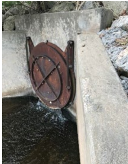
1, 2. Back-flow prevention flap before addition of new features is at left; below with strongback beam and handwheel added to apply pressure to the flap. Slip-resistant grating and handrails allow safe, convenient access
