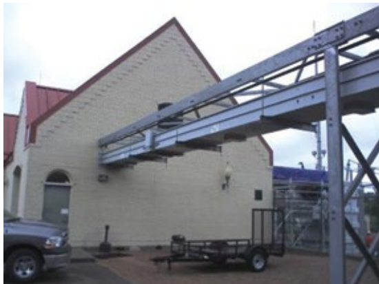
1. Two electrical faults occurred on this section of 13.8-kV bus duct within five years
