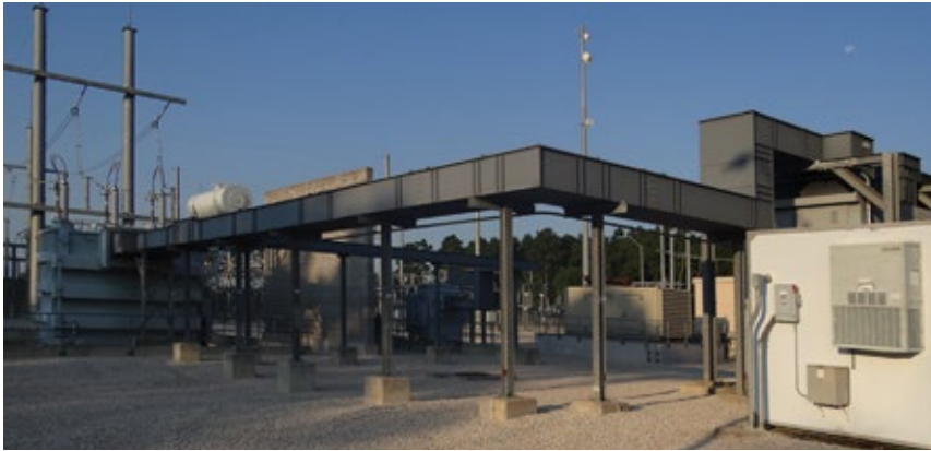
15. Rectangular bus contributed to plant unavailability and was replaced with the circular non-seg shown in Figs 2 and 3
