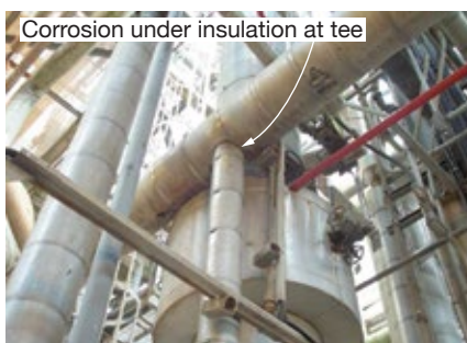
1. Atmospheric corrosion of carbon and low-alloy steel is hidden under insulation
