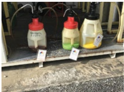
4. Color coding of both oil storage containers and fill ports on equipment (yellow, right) helps to identify a specific lubricant and avoid cross contamination through misapplication
