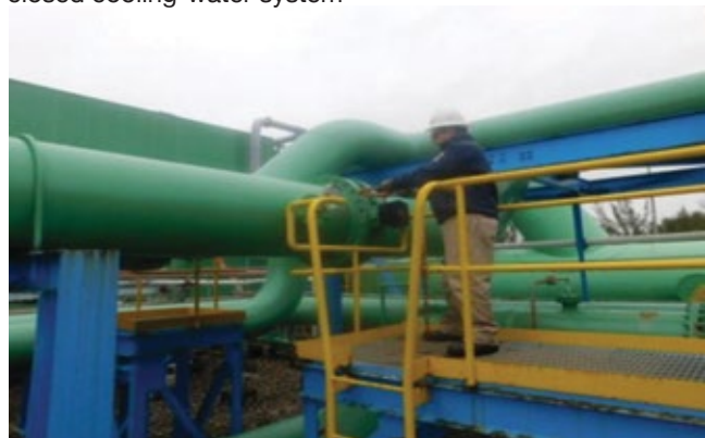
4. Closing heat exchanger’s seawater inlet valve
