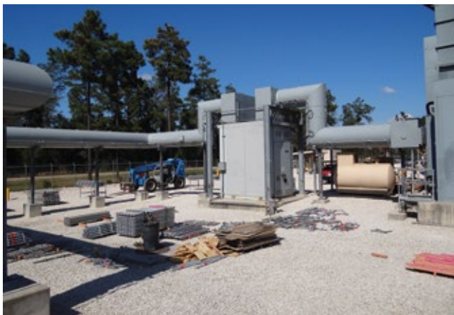
13, 14. Replacement non-seg runs from the generator (extreme right) to the circuit breaker at the center of the left-hand photo; it is shown entering the generator step-up transformer in the right-hand photo
