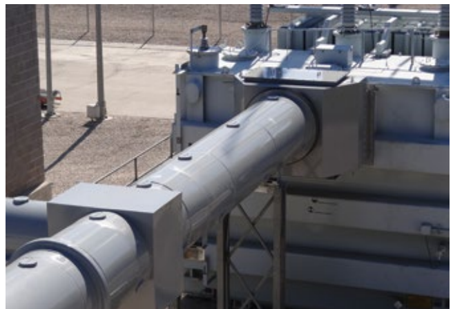
13, 14. Replacement non-seg runs from the generator (extreme right) to the circuit breaker at the center of the left-hand photo; it is shown entering the generator step-up transformer in the right-hand photo
