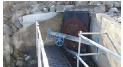
1, 2. Back-flow prevention flap before addition of new features is at left; below with strongback beam and handwheel added to apply pressure to the flap. Slip-resistant grating and handrails allow safe, convenient access
