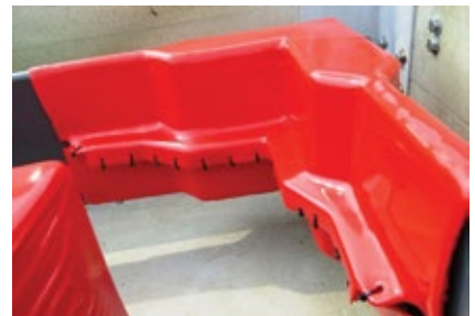
4. New-design insulating boots have tie-wraps at the sides rather than on top
