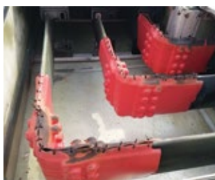
1. Two electrical faults occurred on this section of 13.8-kV bus duct within five years
