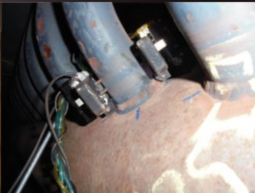
Tube to Header Weld Examination for Cracking
