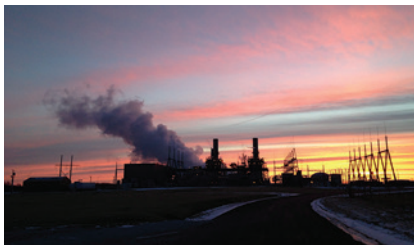
State Line Power Station
