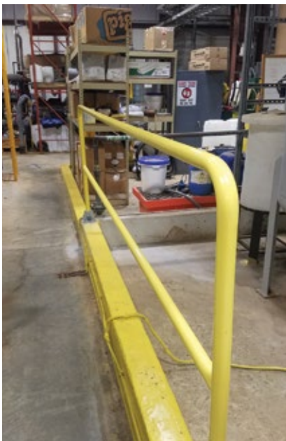
1. Guardrail protects against curb trip hazard
