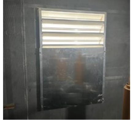
1. Natural ventilation to atmosphere is provided via stationary louvers
