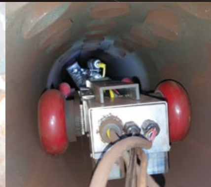
Internal Inspection, Collecting Tube Video & Measuring Wall Loss
