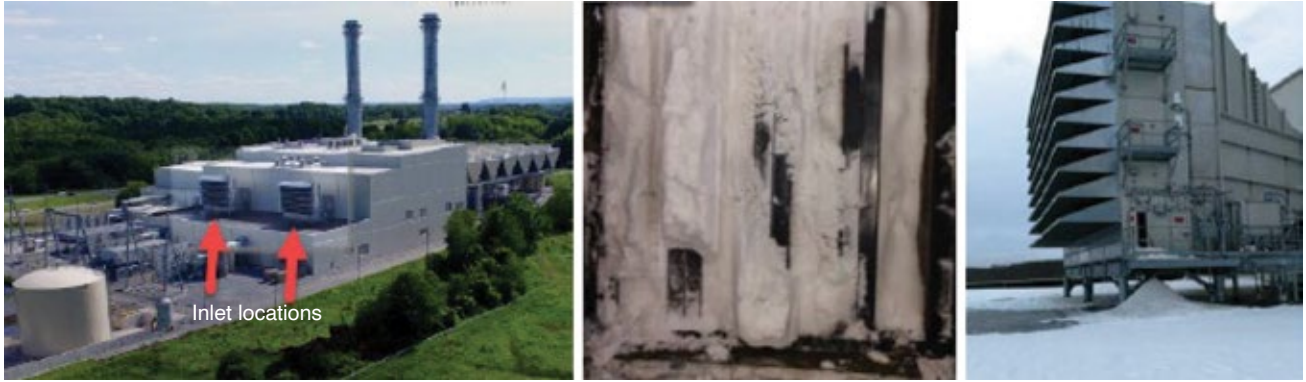
6. Design of the gas-turbine inlet filtration system (left) was conducive to filter plugging (right) during wind-driven snow events (center)
