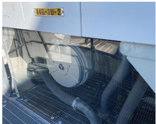
1. A plexiglass panel was installed on the breaker to protect against inclement weather
