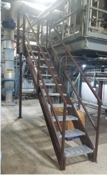
4. Stairs replaced ladder
