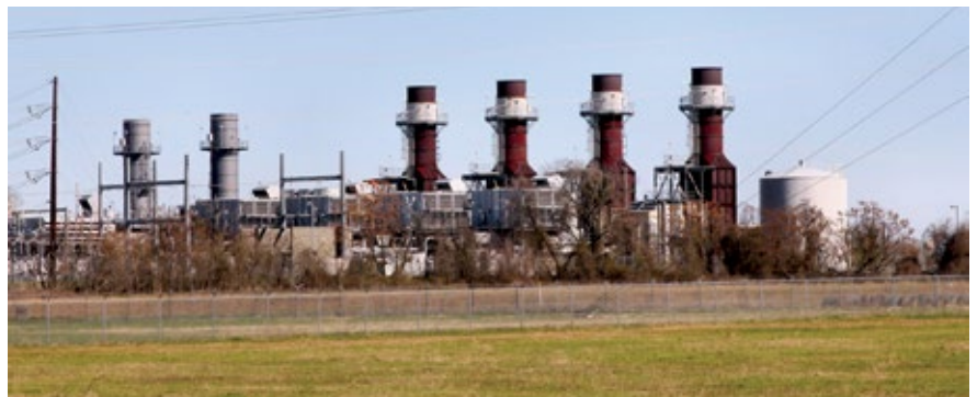
2. Austin Energy’s Sand Hill Energy Center was erected in stages: four simple-cycle LM6000s in 2001, a 300-MW 1 × 1 combined cycle in 2004, and two simple-cycle LM6000s in 2010. Total generating capability is 595 MW
