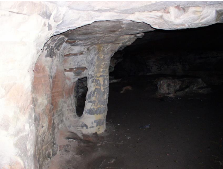
Left: One of the pillars left close to the side wall of the chamber.
