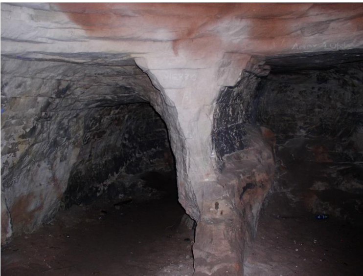
Left: Side alcoves and supporting pillars. Soot deposits can be seen on the walls from campfires.
