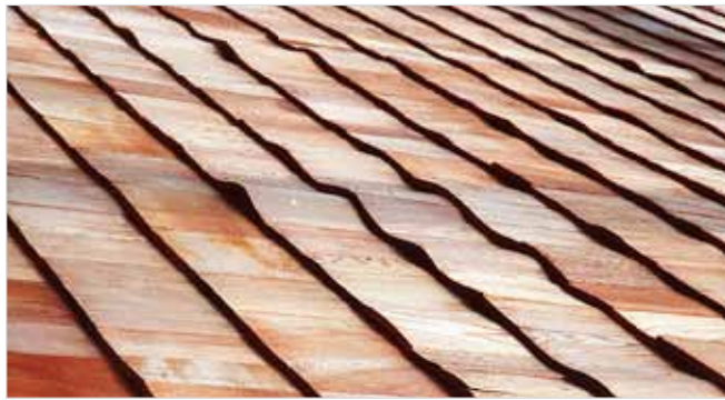
Figure 5. Buckling of shingles installed with insufficient space between adjacent shakes/shingles to accommodate swelling.
