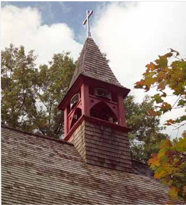
Figure 4. Thirteen-year-old shingle roof with random-width shingles.
