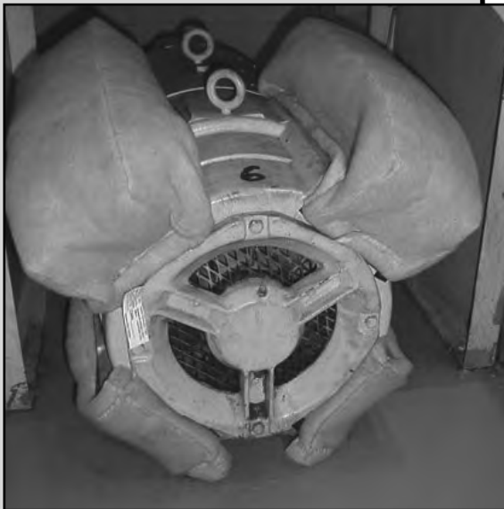
NEW CLEAN INSTALLATION (IMPERIAL 366)
