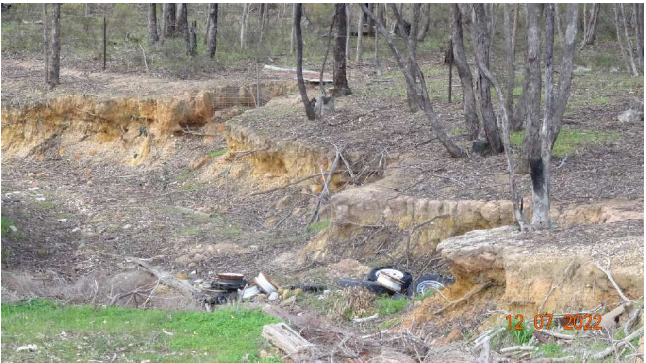
Close of photo of the gully. Although it can be sometimes beneficial to batter a gully (smooth off the eroding sides) to assist with rehabilitation. However, there is the chance there could be existing holes or hollows in the bank of the gully which may provide habitat to nesting Pardalotes or Rainbow Bee-eaters. Therefore, it is not recommended to batter the gully.
