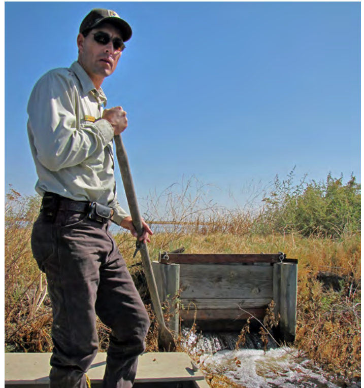
Manager checking a water control structure at Twin Lakes Partners for Fish and Wildlife project - Shawn Milar
