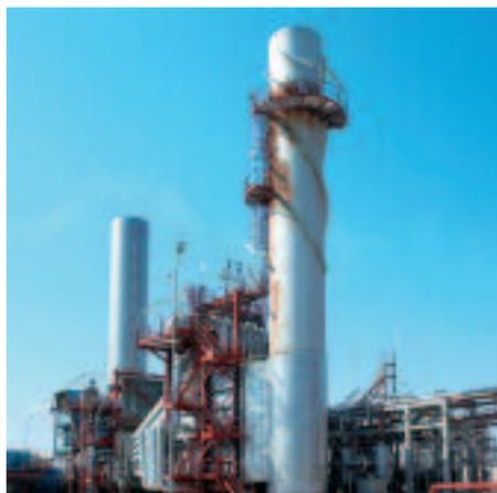
NUEVA GENERADORA DEL SUR (a 50/50 joint venture between CEPSA and UNIÓN FENOSA) operates a natural gas-fired combined cycle power plant located on the premises of CEPSA's "Gibraltar" Refinery, with two power generating sets, having an overall output of 780 MW according to the Guaranteed Output Tests.
