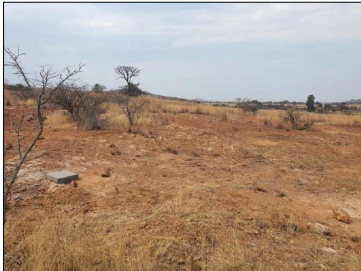
Figure 4-3: View of cleared and excavated surfaces at the proposed quarry site .
