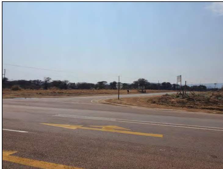
Figure 4-1: View of general surroundings at the R516 – R511 intersection, the western offset of the project.
