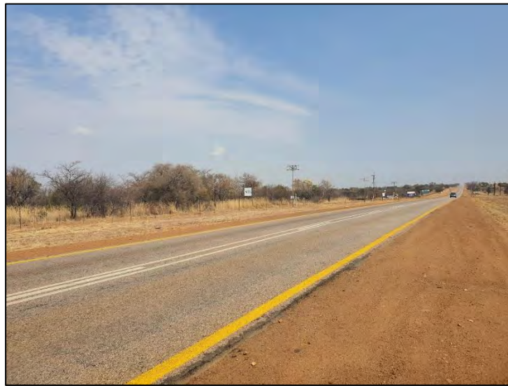
Figure 4-6: View of general surroundings along the SANRAL servitude in the project area looking west.
