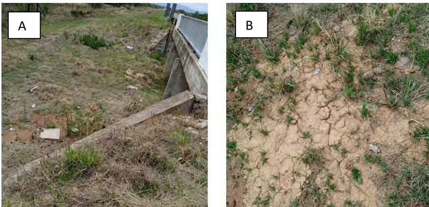
Plate 4: Images of the watercourse at Bypass B3227. A) The servitude was mainly grass covered with dominant clay B) Soils in this area were mostly clay soils.
