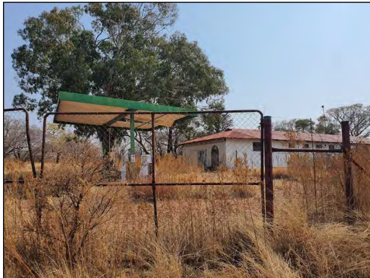
Figure 4-12: View of an old store and filling station along the R516 road, outside the road servitude.
