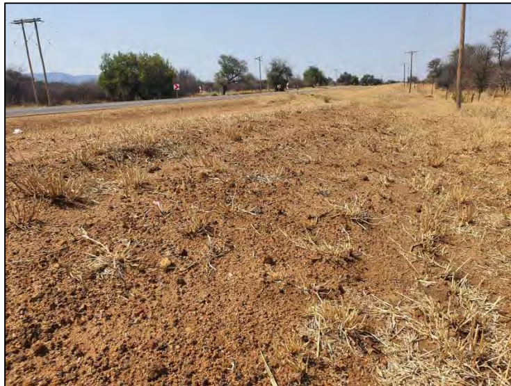
Figure 4-9: View the R516 road servitude in the proposed project area..
